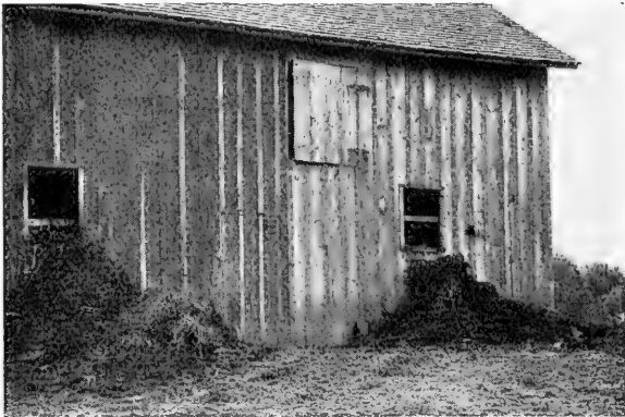
FIG. 44.—A poor way to store barnyard manure, even when the ground is level. The barn is badly rotted by this method. (Animal Industry.)
